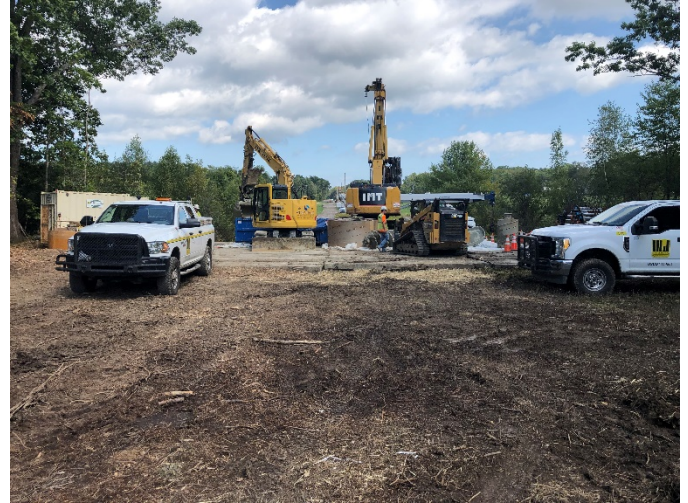
Fig 30: Drilling at Str. 106. Viewing east. (9-11-19).
