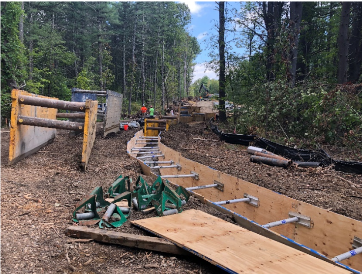
Fig 27: Trenching towards Str. 100. Viewing southeast. (9-11-19).
