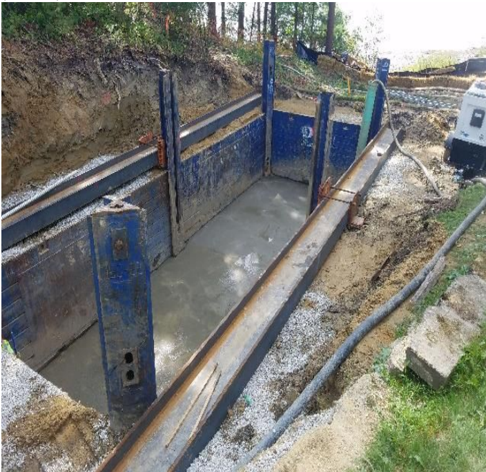
Fig 3: Mud slab poured in man hole at Gundalow Landing. Viewing west. (9-05-19).
