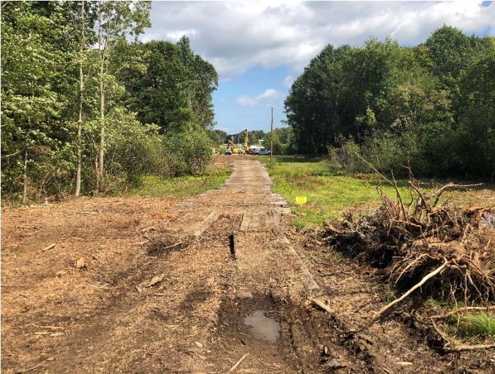
Fig 29: Matting towards Str. 106. Viewing east. (9-11-19).
