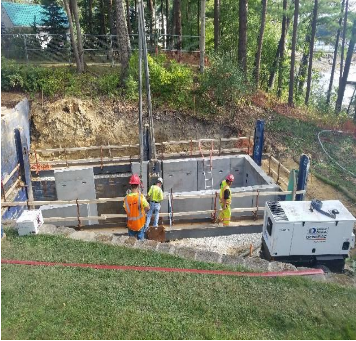
Fig 13: Assembling manhole at Gundalow. Viewing south. (9-9-19).
