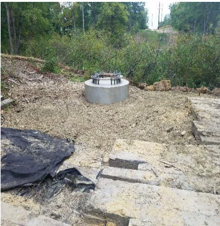
Fig 23: Str. 28 foundation. Viewing north. (9-10-19).
