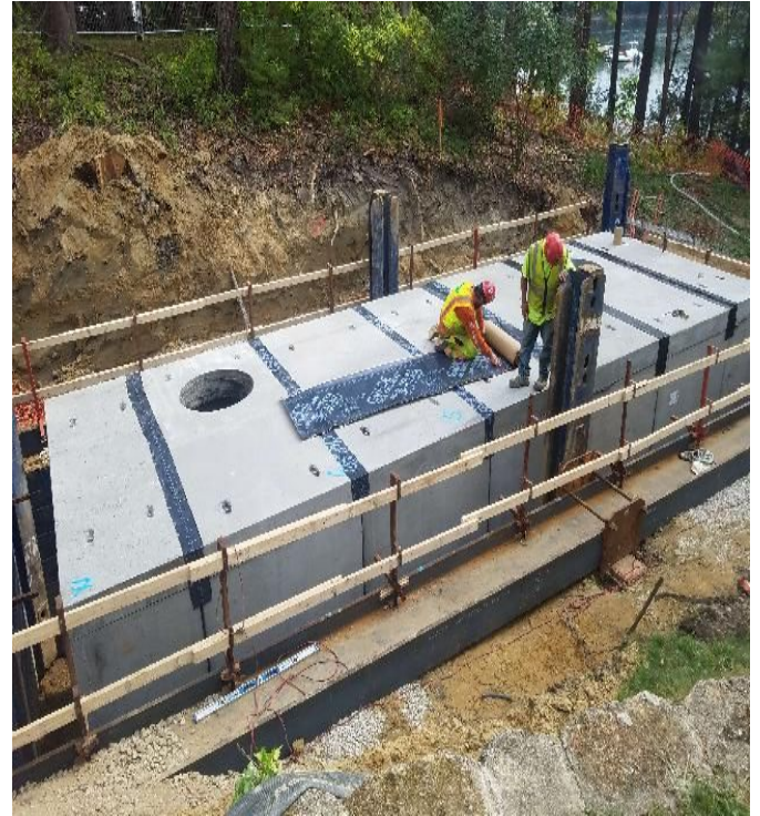
Fig 26: Continuing to assemble manhole at Gundalow Landing. Viewing southeast. (9-10-19).
