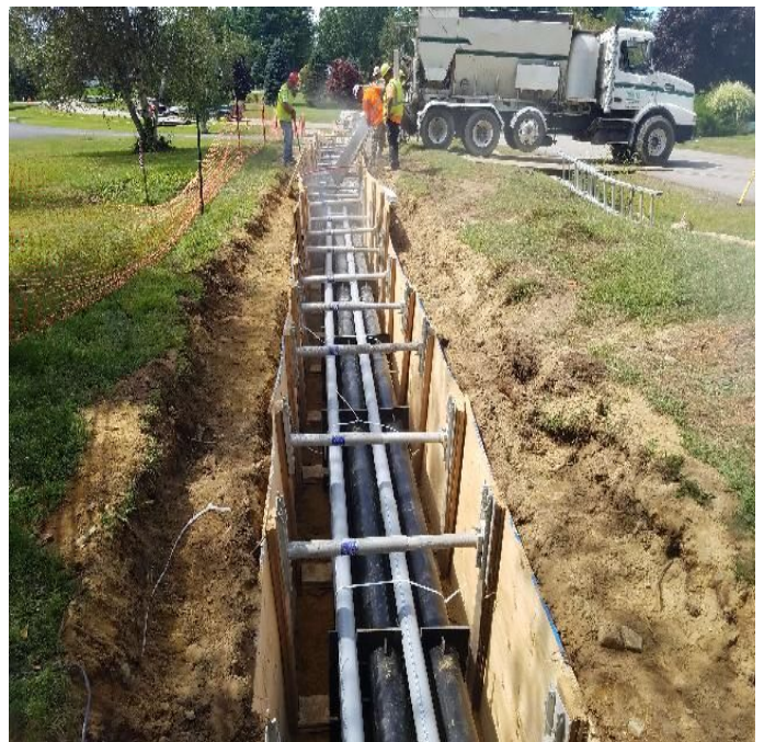
Fig 4: Pouring duct bank along Gundalow Landing Rd. Viewing west. (9-05-19).
