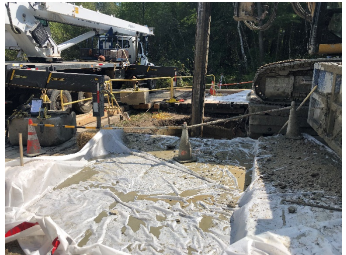
Fig 32: Closer view of drilling at Str. 106. Viewing south. (9-11-19).
