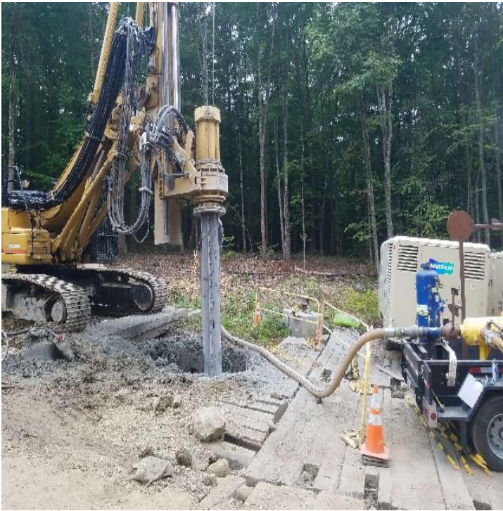
Fig 21: Drilling Str. 29. Viewing west. (9-10-19).
