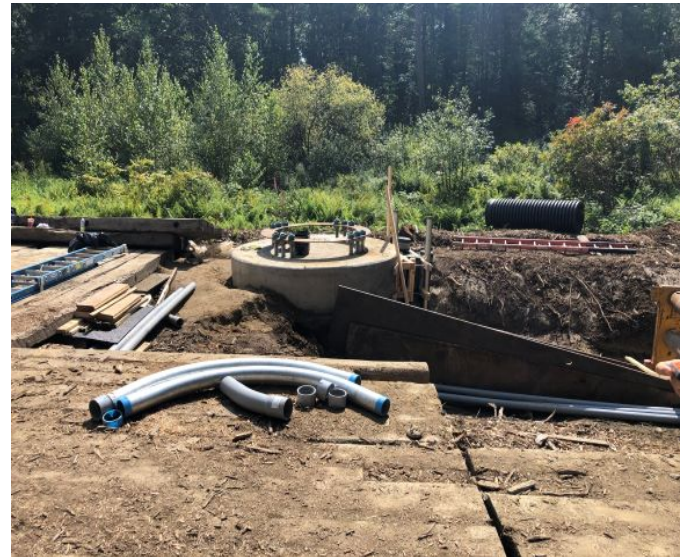
Fig 28: Str 100. Viewing south. (9-11-19).
