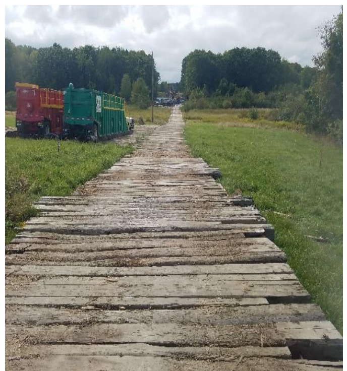
Fig 24: Matted access road leading to Str. 106. Viewing southwest. (9-10-19).
