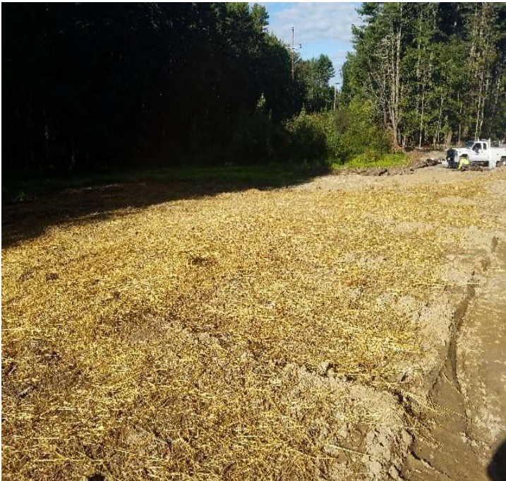
Fig 9: Straw broadcast over soils spread out in the uplands near Str. 100. Viewing southwest. (9-9-19).
