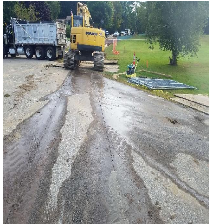
Fig 18: Prepping to trench across Gundalow Landing Rd. Viewing east. (9-10-19).
