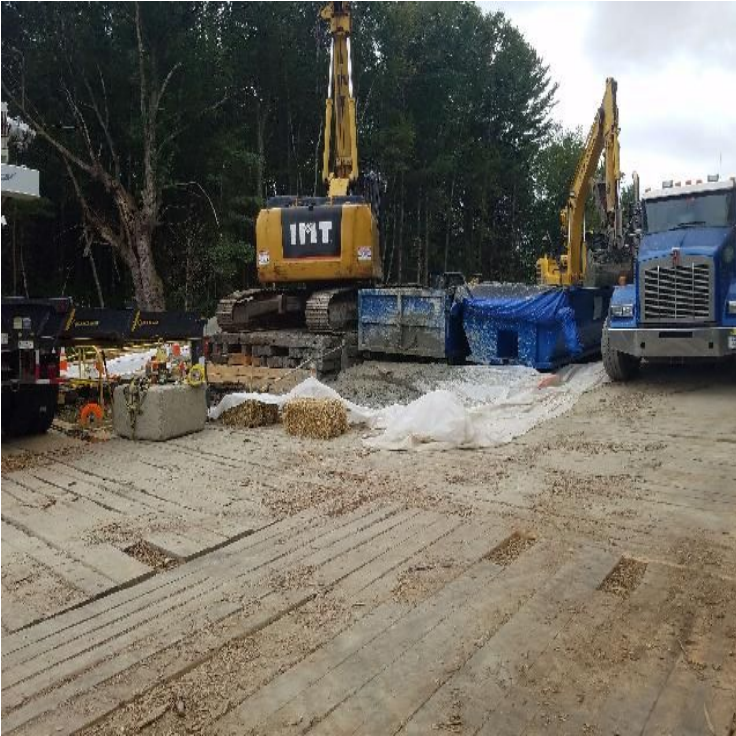
Fig 25: Drilling Str. 106 and containerizing soil spoils. Viewing southwest. (9-10-19).
