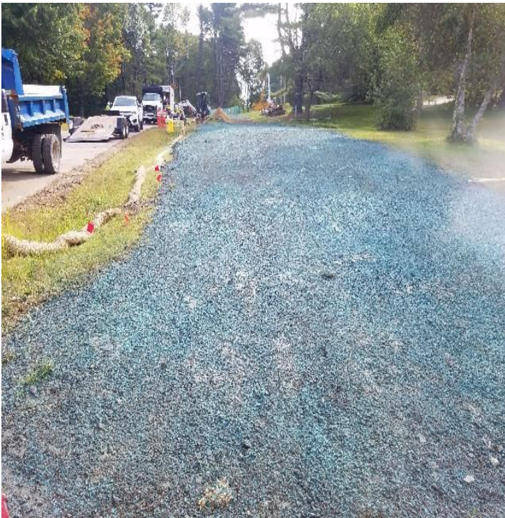
Fig 19: Restored trench area at Gundalow Landing hydro seeded. Viewing east. (9-10-19).
