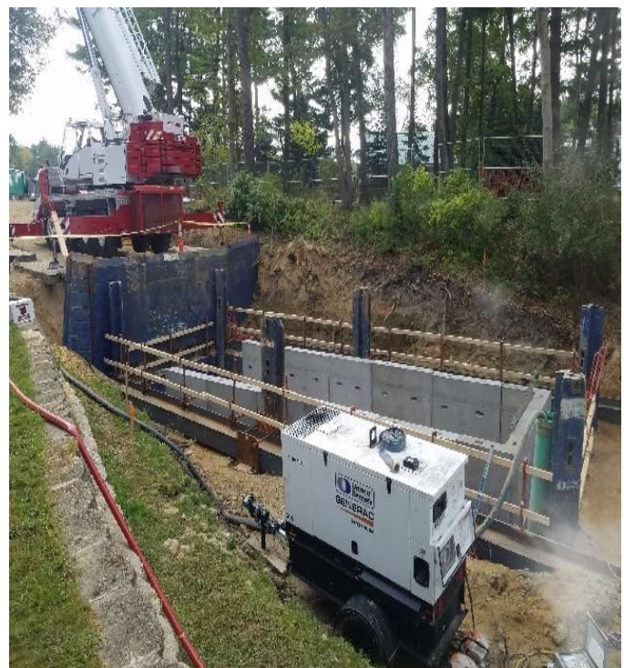
Fig 16: Assembling manhole at Gundalow Landing. Viewing southeast. (9-10-19).
