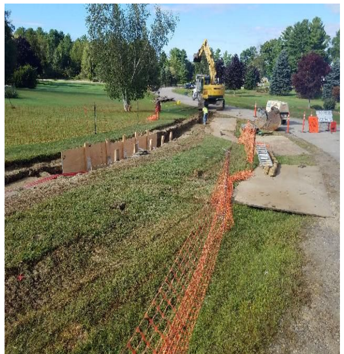
Fig 12: Continuing to excavate duct bank along Gundalow Landing Viewing west. (9-9-19).
