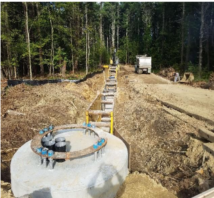
Fig 7: McCourt trenching from Str. 100 towards Gundalow Landing. Viewing west. (9-6-19).
