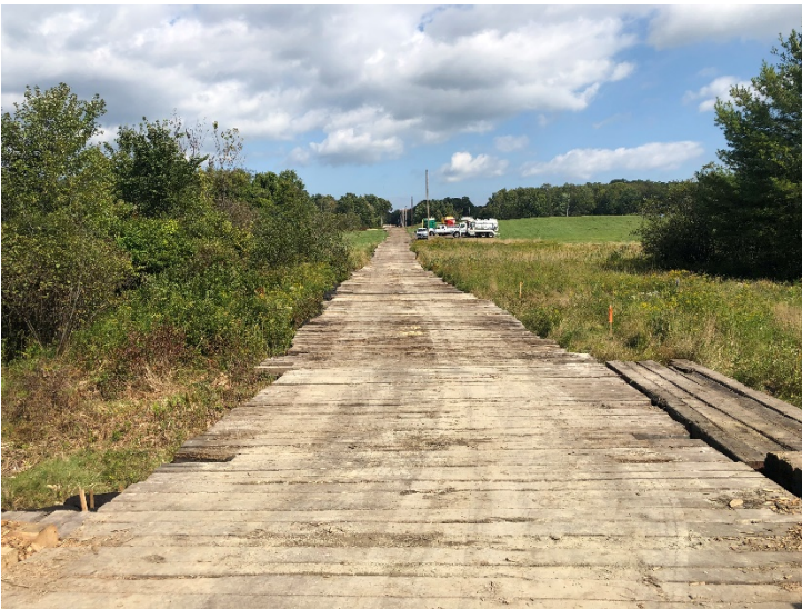
Fig 31: Matting across wetland and stream east of Str.106. (9-11-19).
