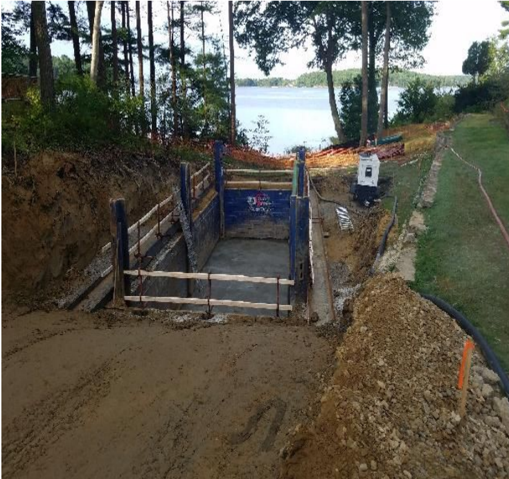
Fig 5: Mud slab poured in man hole at Gundalow Landing. Viewing southwest. (9-6-19).
