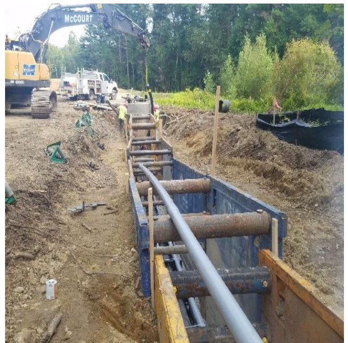
Fig 10: Trenching activities continue from Str. 100 to Gundalow Landing. Viewing north. (9-9-19).
